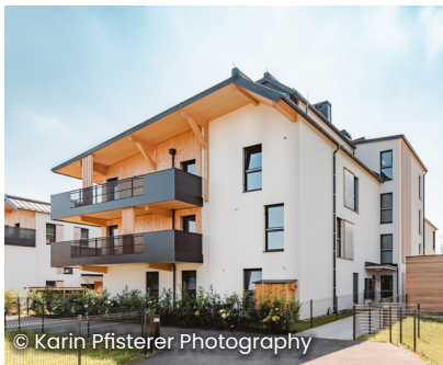
© Karin Pfisterer Photography This development by Siges Massivholzbau, comprises 80 apartments. 3,000 m 3 of wood, partly sourced from local PEFC-certified forests, was used in its construction, making it one of the largest multi-story wooden residential buildings in Salzburg, Austria.
