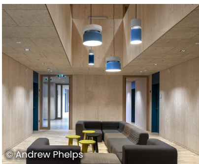
© Andrew Phelps The Wood Technology Association boarding school in Kuchl, Austria, used over 1,000 m 3 of CLT, supplied by Mayr-Melnhof in its construction.
